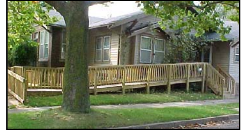
Handicap Ramp built in Waterloo
